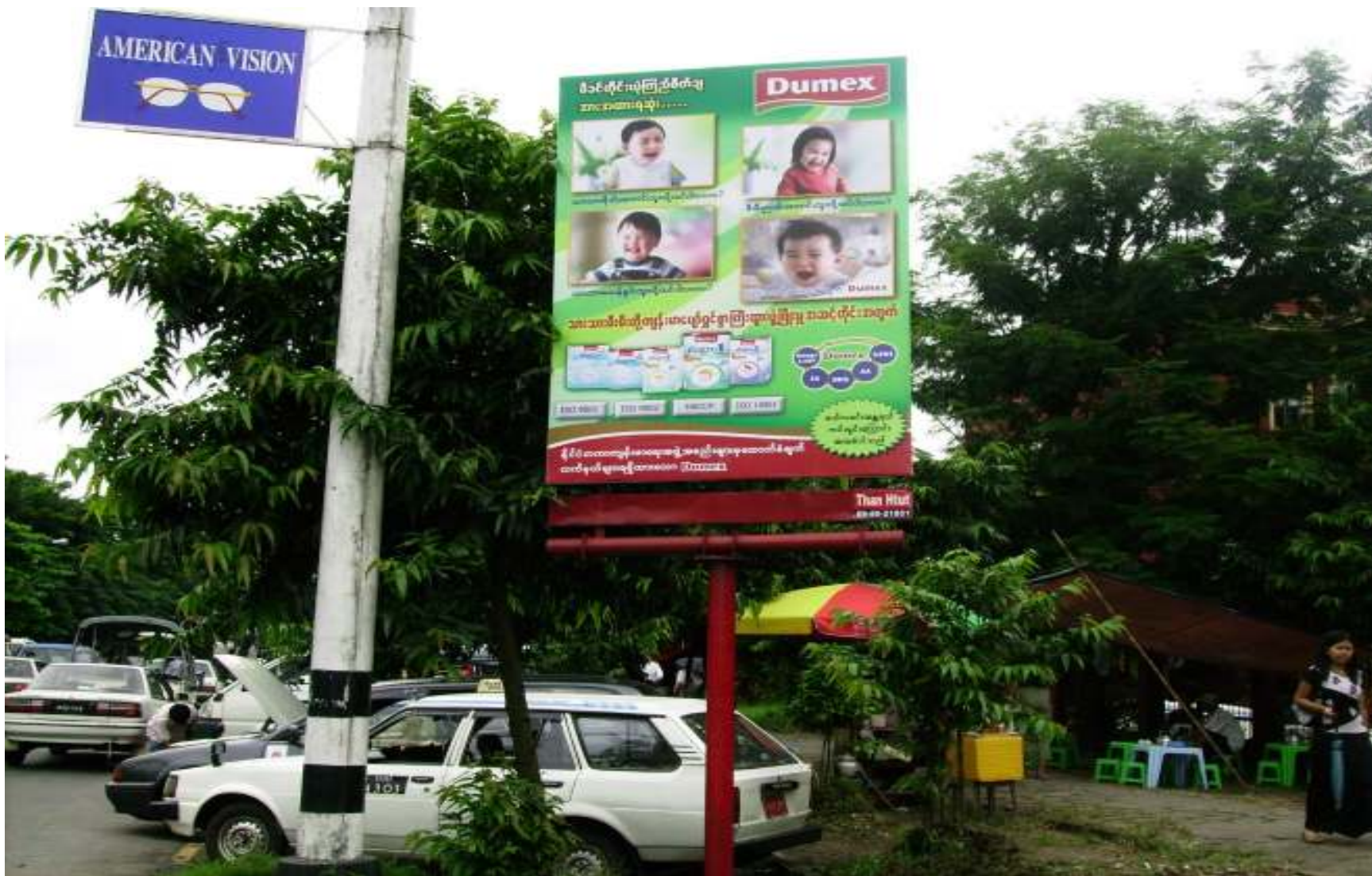
Erecting of bill board in public place near entrance of Zoo
